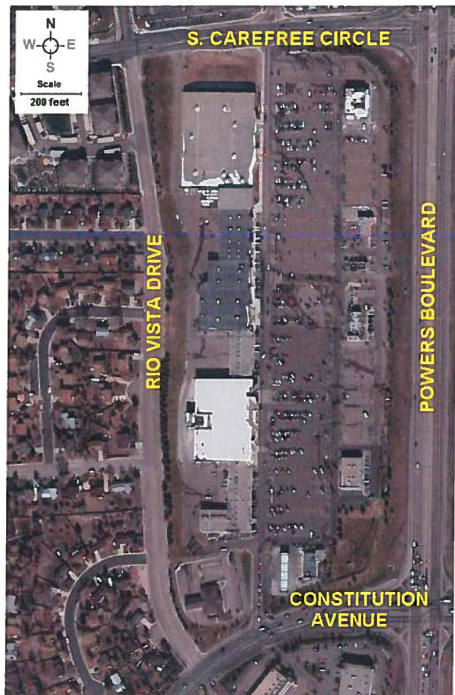
Exhibit 5-5. Aerial View of Rio Vista Drive between South Carefree Circle and Constitution Avenue
